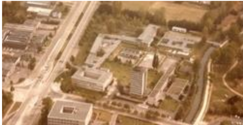
Figure 1. Aerial photograph of the late-1950s building, flanking Hasselt's outer ring road to the North. Credits and date unknown
